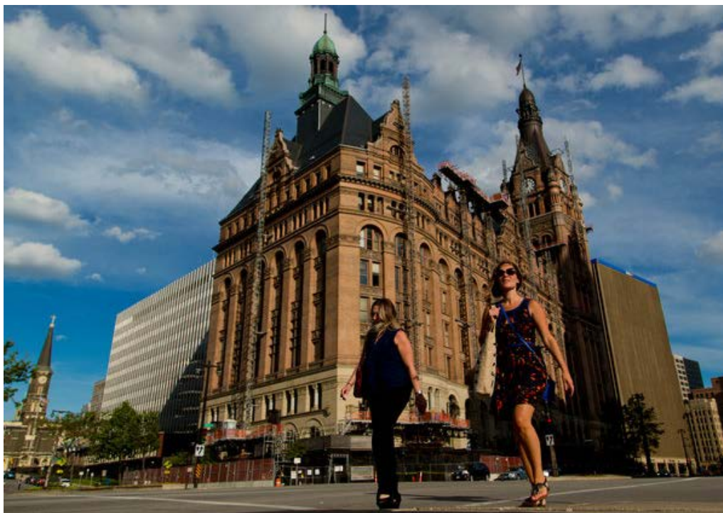
The Milwaukee City Hall, below, was built more than 100 years ago on a wooden foundation. Darren Hauck for The New York Times
