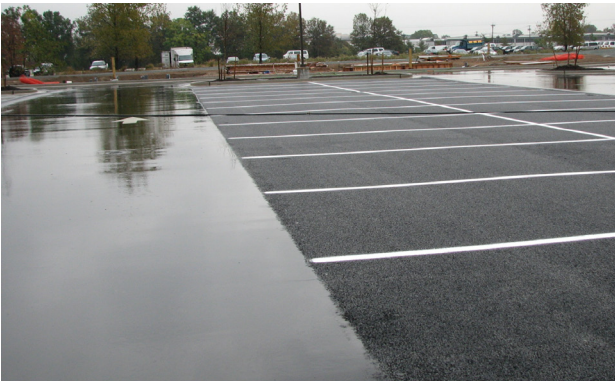
Figure 4. Traditional asphalt (left) and porous asphalt (right) during a rain event. The traditional asphalt looks wet and shiny, while the porous asphalt surface is relatively dry.
