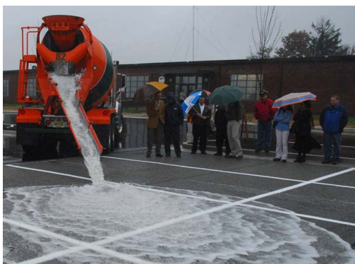
Figure 1. A cement truck discharging 2,000 gallons of water onto a permeable pavement. The water was drained from the surface in less than 4 minutes.
