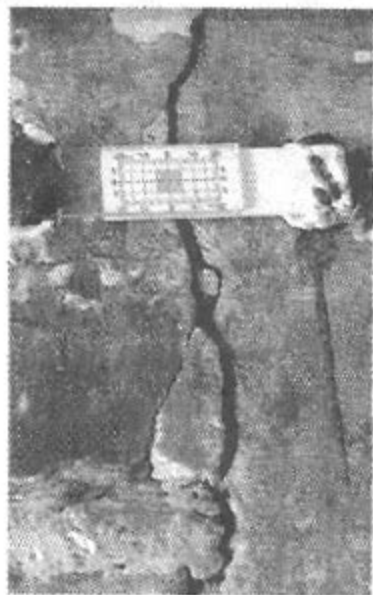
A structural monitoring device is installed in the basement of a building on Hemenway Street.
